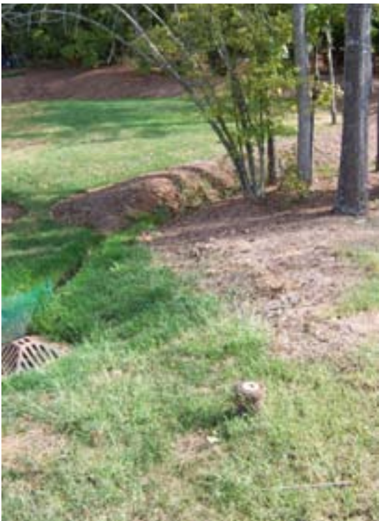
Photo 7 – Looking “upstream” along side drainage ditch on private property.
