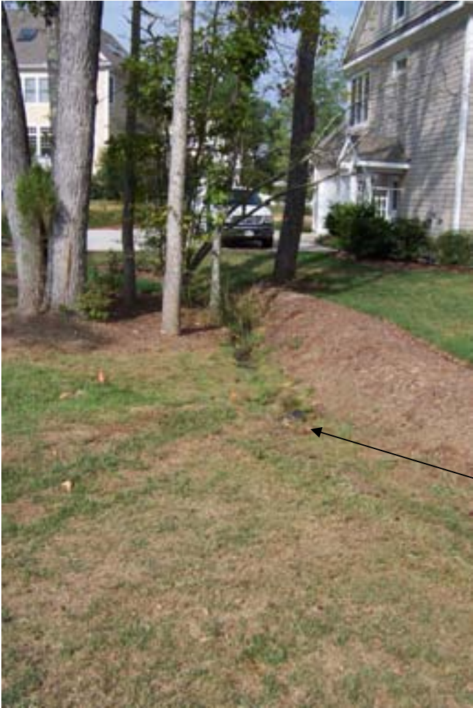
Photo 3 – Roof drain outlets from 412 and 410 Simerville Rd at side drainage ditch.
