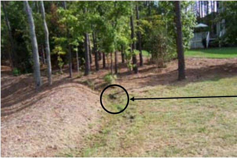
Photo 5 – Roof drain outlet from 408 Simerville Rd home.
