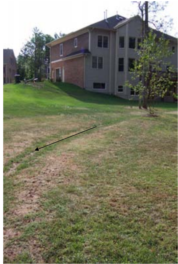
Photo 2 – Arrow indicates location of roof drain lines from 412 and 410 Simerville Rd, across Ms. Brown’s property.
