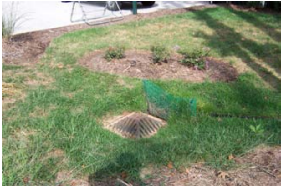
Photo 8 – Yard inlet at terminus of side drainage ditch
