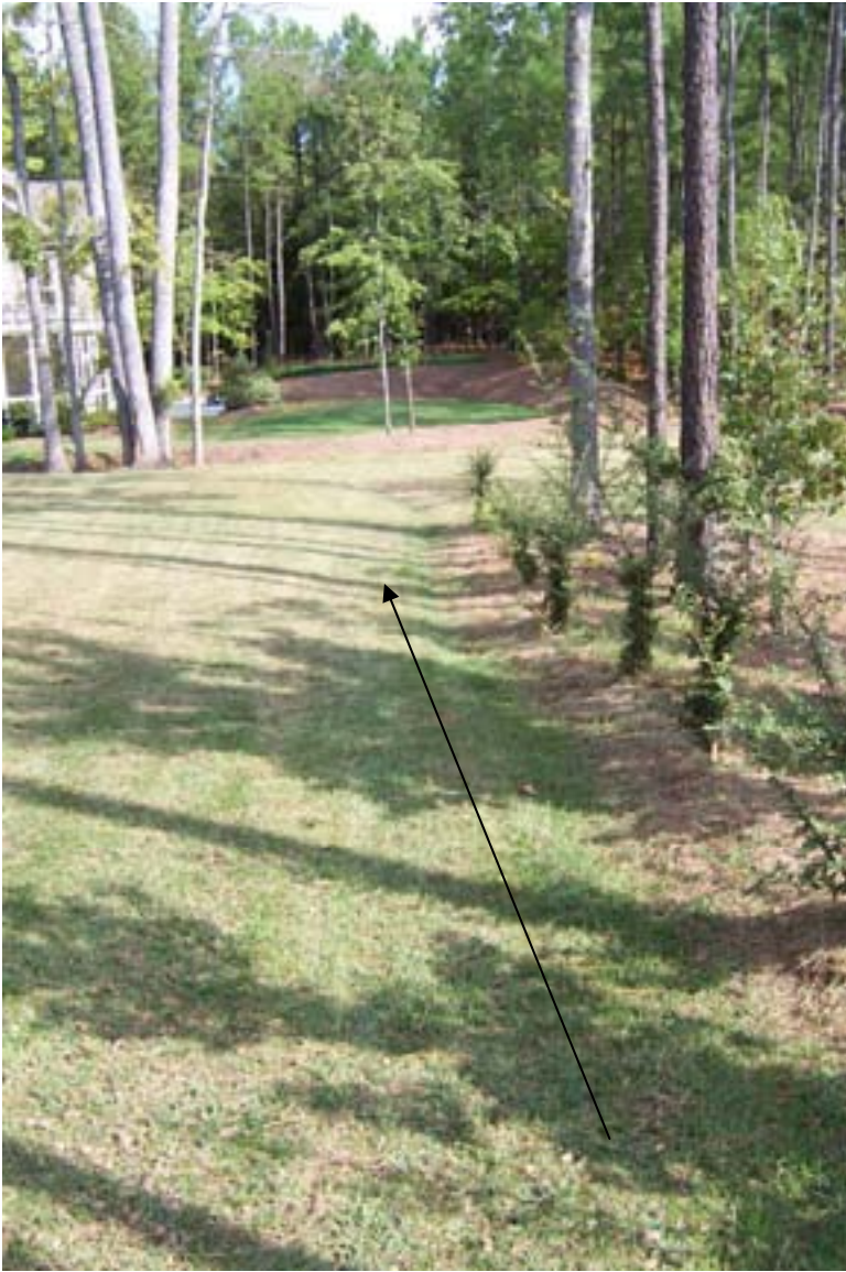
Photo 1 – Looking toward side drainage ditch along a drainage swale in Ms. Brown’s yard. Arrow indicates direction of drainage. Roof drain lines from homes at 412 and 410 Simerville Rd come in from right, just past the natural area.
