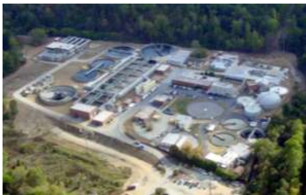
The Mason Farm Wastewater Treatment Plant (WWTP)
