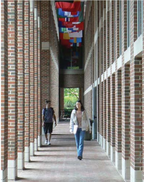
McColl Building, University of North Carolina at Chapel Hill
