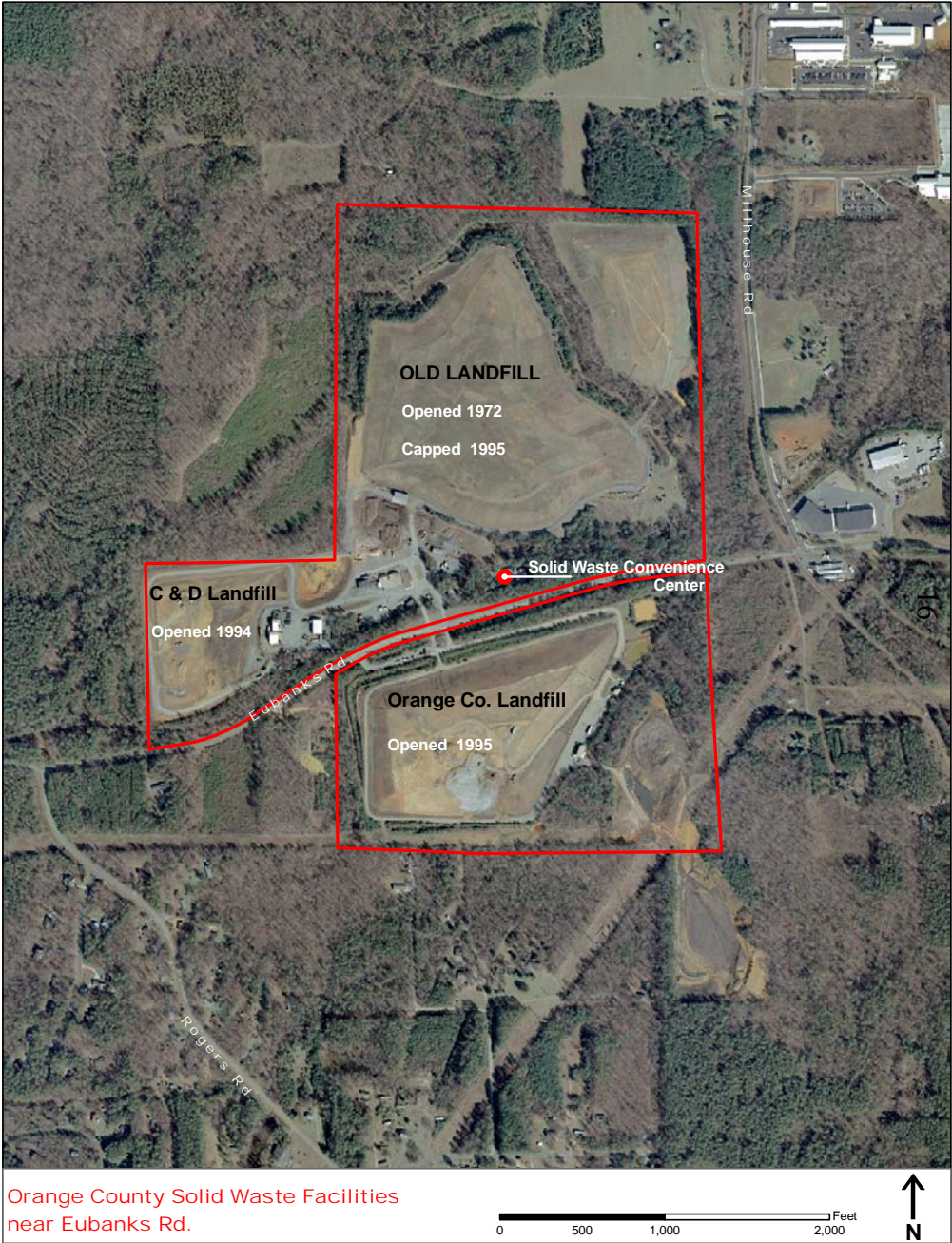
Figure 3 - Aerial Image of Orange County Landfills
