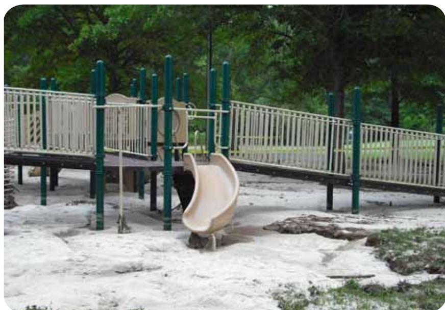
Image of flood damage after Hurricane Hannah during the summer of 2008. Photo courtesy of the Town of Chapel Hill.
