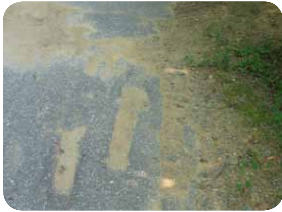
1 The length of the corridor has vegetation encroaching the edges of the trail's surface and causing the trail to crumble and crack. Sediment is also an issue due to clogged drainage pipes. The surface condition of the asphalt paving is fair, except for damaged areas such as the equipment damage shown above.
