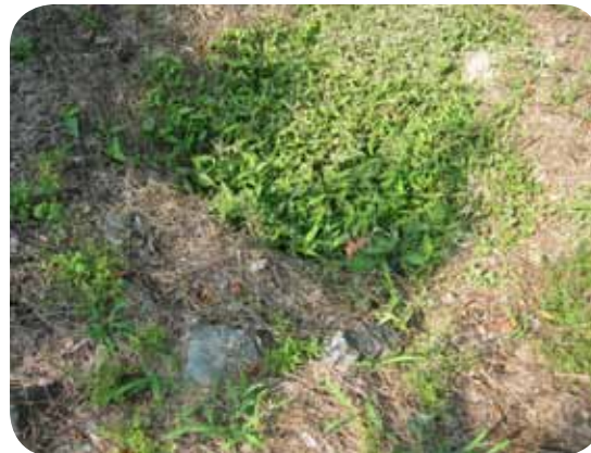
2 Clogged drainage pipes and culverts are increasing flood-related issues along this trail, including the deposits of sediment and leaf litter along the trail's surface.
