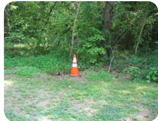
5 Large ruts, holes from uprooted trees, and animal dens should be filled in along the trail corridor to prevent a potentially hazardous situation for trail users and maintenance vehicles.
