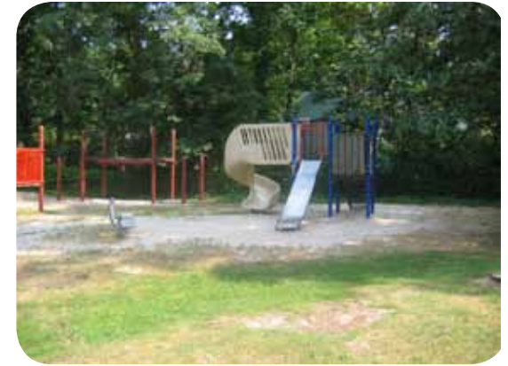
3 The safety surfacing needs to be removed and replaced with engineered wood fiber or poured-in-place rubber surfacing. Edging should be installed to ensure adequate safety surfacing remains within the fall zone.
