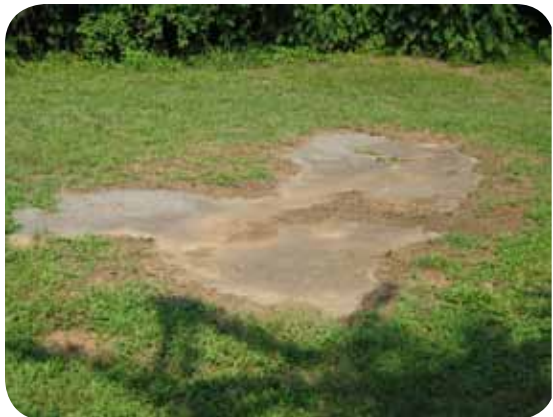
4 Areas such as this pavement should be removed from the greenway corridor, particularly since it is in the floodway of Bolin Creek. Pavement such as this is not usable, increases the impervious surface within the floodway, and is not aesthetically pleasing.
