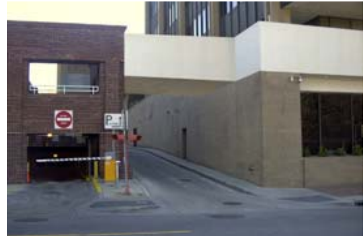
Illustration showing a potential connection from Bank of America plaza to Rosemary Street parking deck.
