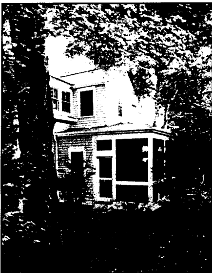
A small rear addition expands the second floor with a central bay and encloses a space behind the screened porch. Like the rear addition on the opposite page, this addition is not visible from the street.
