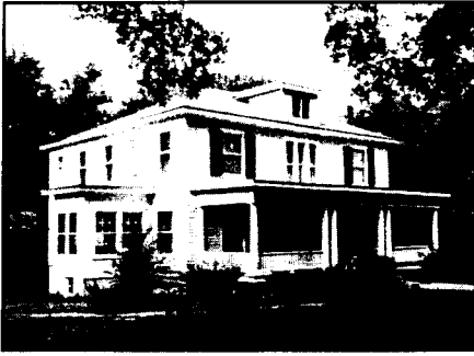
Deteriorated elements of this front porch were replaced in kind during rehabilitation.
