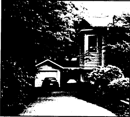
The roof of this one-bay garage was extended to provide shelter for a second vehicle.
