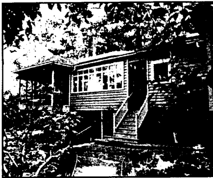
A small one story addition connects a new screened porch with the original house along the rear elevation of this district house.
