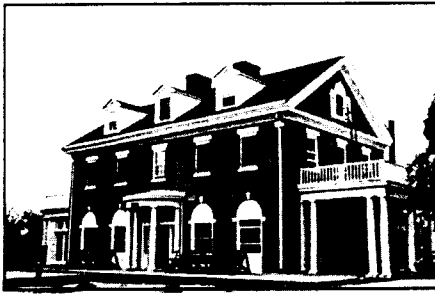
Many well-detailed brick residential properties are found within the historic districts.
