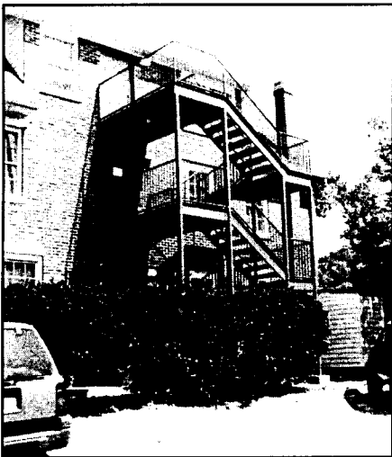
This steel firestair was located on the building's rear elevation, painted in a color to blend with the brickwork, and screened at its base with shrubbery.
