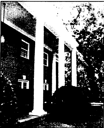
The wooden columns, soffit and cornice of this two story portico were carefully repaired and restored.
