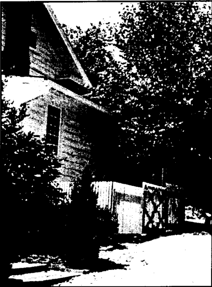
Above, a small section of wooden picket fencing visually screens the outside mechanical units from view.
