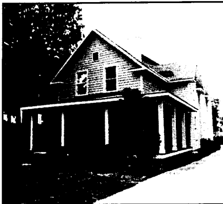
A substantial rear addition to this district building repeats the form of the original house without enlarging the front facade as it extends the depth of the building.
