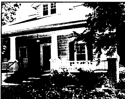
Six-over-one doublehung window sashes replaced inappropriate fixed single-pane glass panels during the sensitive rehabilitation of this bungalow.
