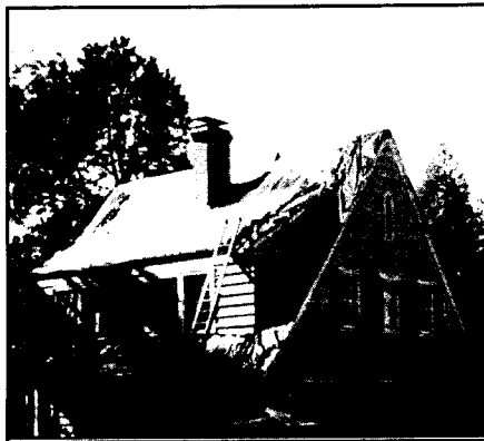
Above, deteriorated roofing shingles on this prominent, steeply-pitched roof are being replaced with new shakes that resemble the original roofing treatment.
