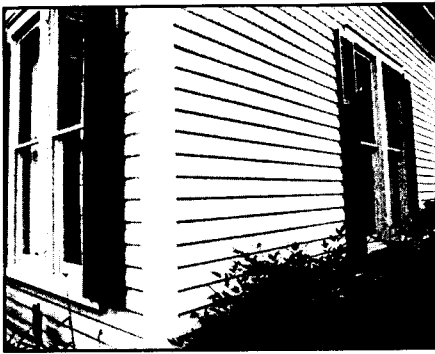
German siding with traditional trimwork wraps the exterior of this frame house.
