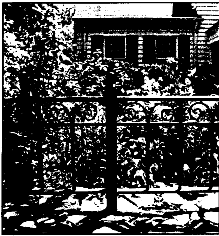
This low cast iron fence with decorative wrought iron inserts tops the fieldstone wall bordering a front yard.
