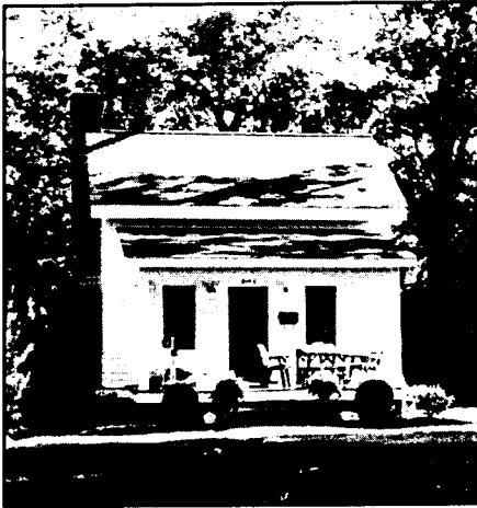
The Andrews house on its new foundation after relocation.
