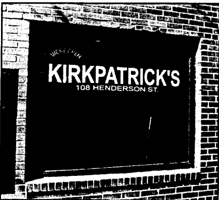
Opaque lettering applied directly onto display windows is an effective, economical, and easily reversible form of signage that is appropriate within the historic districts.
