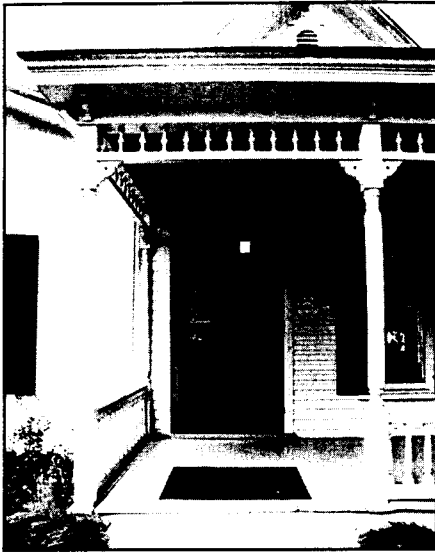
The turned columns, decorative spindlework, brackets, and turned balusters of the porches above and opposite illustrate the versatility of wood to be milled in a variety of forms.
