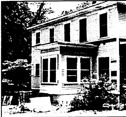
Above, deteriorated wooden weatherboards are selectively replaced in kind to match existing siding during rehabilitation.
