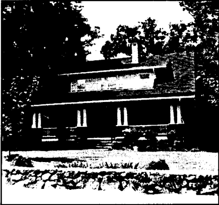
The fieldstone foundation and column bases of this frame bungalow repeat the pattern and texture of the low fieldstone walls that wrap so many streetscapes throughout the historic districts.
