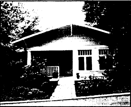
During rehabilitation the front porch of this bungalow, which had been fully enclosed earlier, was partially reopened.
