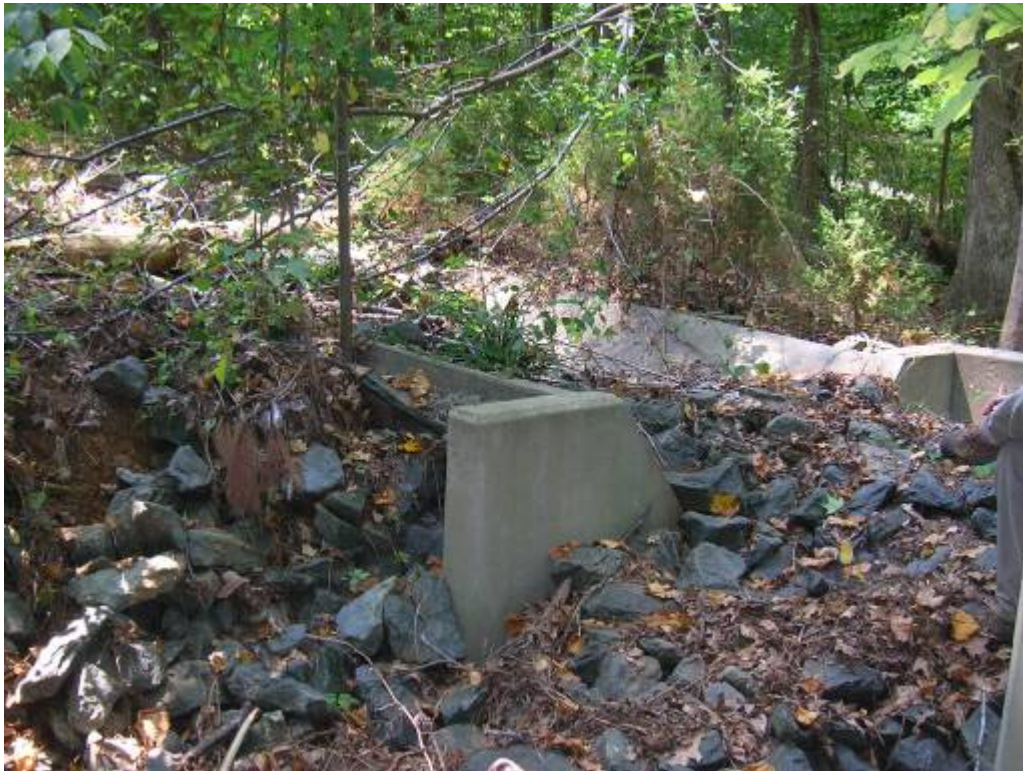
The concrete flow dissipation structure at Site 4.
