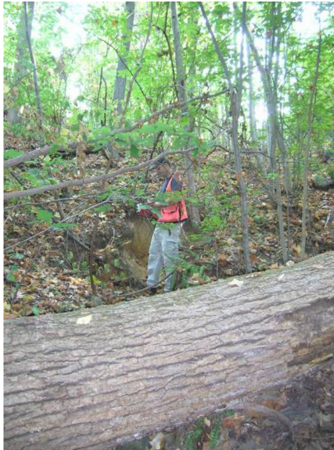
Flow from the stormwater outfall is causing hill erosion before flowing into the existing BMP. Facing northeast.
