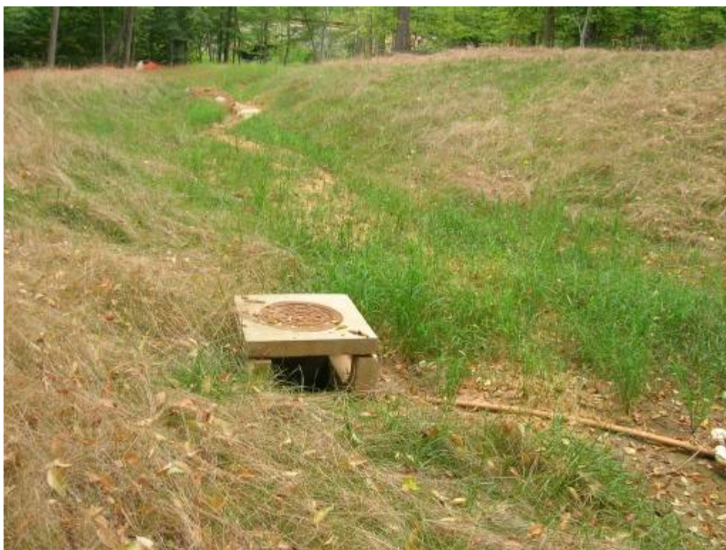
Another sediment basin at Site 6. Note the eroding grassy swale leading into the basin. Facing east.
