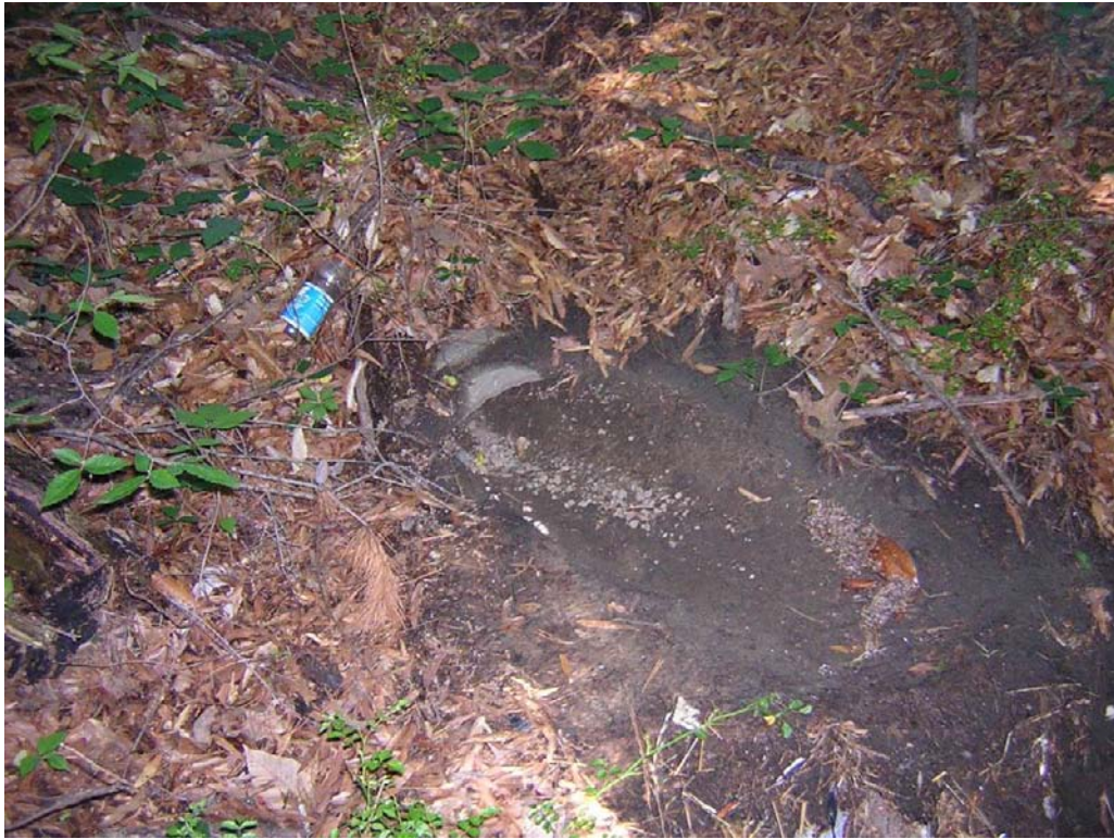
The stormwater outfall pipe from Hillsborough Street is almost completely buried. Facing northwest.
