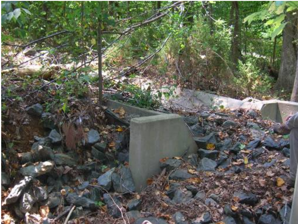
The concrete flow dissipation structure at Site 4.
