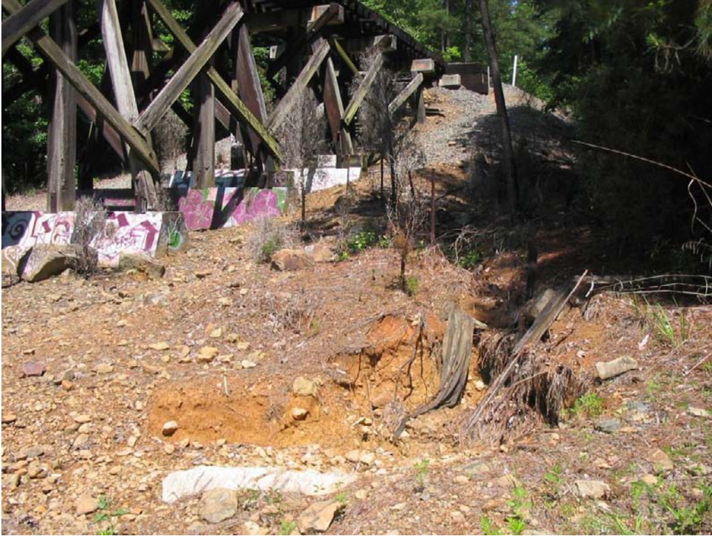
A view of the erosion occurring adjacent to a railroad trestle. Facing north.
