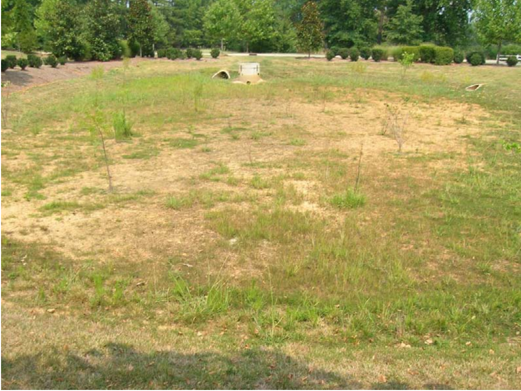
The existing stormwater basin. Note the lack of vegetation and the close proximity of the inlet pipe to the outlet structure.
