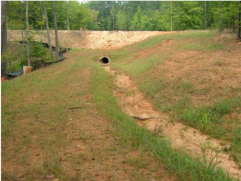
An eroding grassy swale, facing west.
