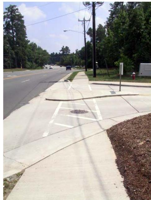
**Diverter intended to restrict left turns at this driveway lacks curb cuts and creates an obstacle for pedestrians.**
