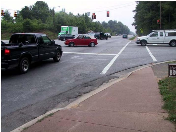
**Single corner curb cut is misaligned with crosswalk at Estes Drive.**
