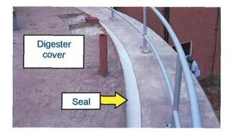
Left: Part of a fixed digester cover structure including the seal installed to prevent leaks at the perimeter of the cover.
