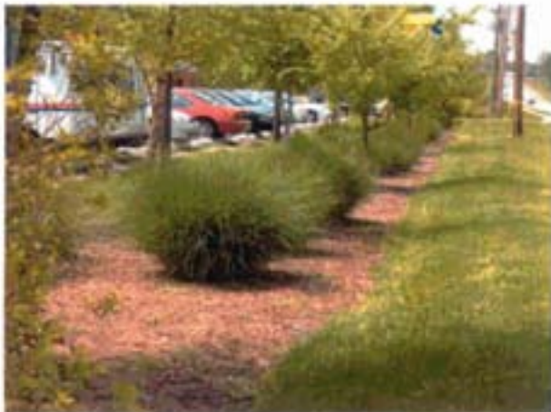
Bio-retention basin in Greensboro, NC Photo courtesy of North Carolina State University — Biological and Agricultural Engineering
