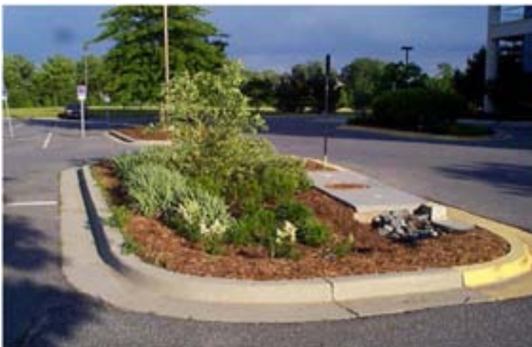
FIGURE 3.2-1 Bioretention in Parking Lot Island
