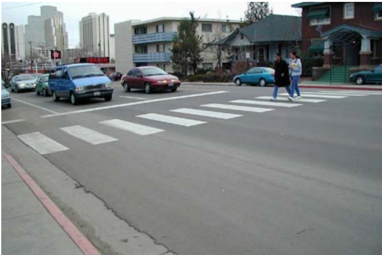
Figure 8. High-visibility crosswalks can make the crosswalk more visible to approaching motorists.
