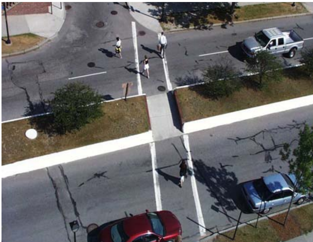
Figure 9. Marked crosswalks alone are not recommended at high-volume multi-lane streets without other substantial pedestrian measures.
