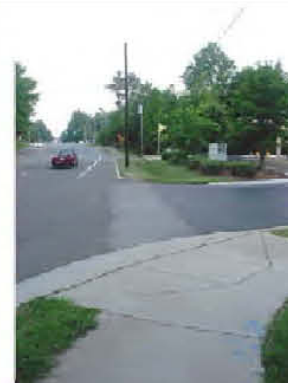
SIDEWALK LACKING PAVED CONNECTION NEAR NORTHFIELD DRIVE
