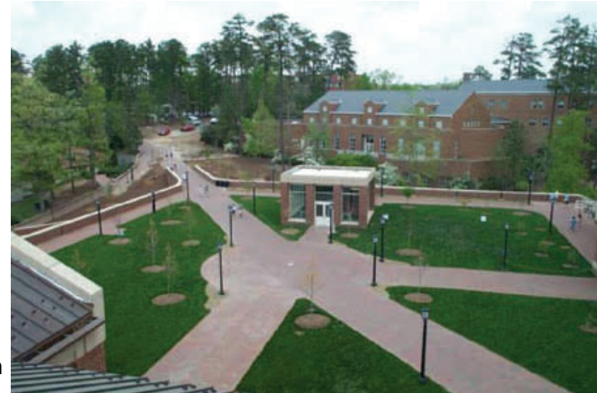
A vegetative roof and cistern on top of the Ram's Head parking garage reduces urban stormwater runoff
