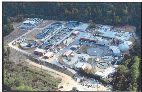
Aerial view of the Mason Farm Wastewater Treatment Plant, October 2007.
