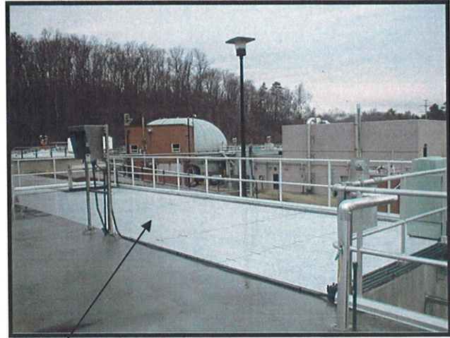
Cover over new headworks structure
