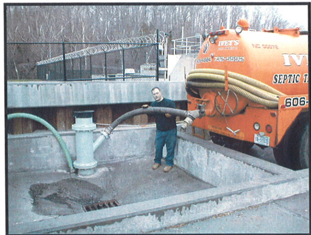
New septage receiving facility
