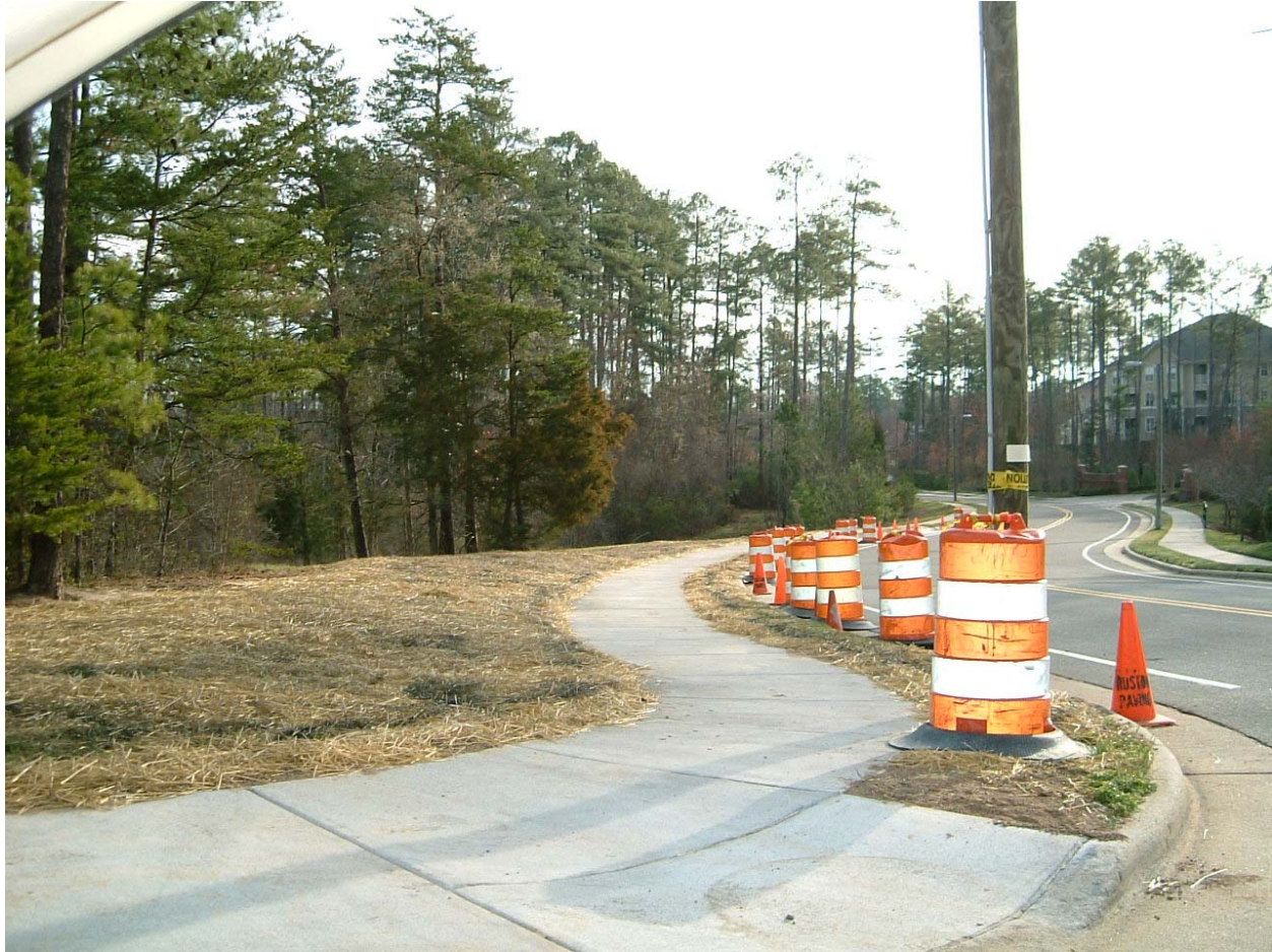
Picture 4b: Partially repaired bus pull-off.
