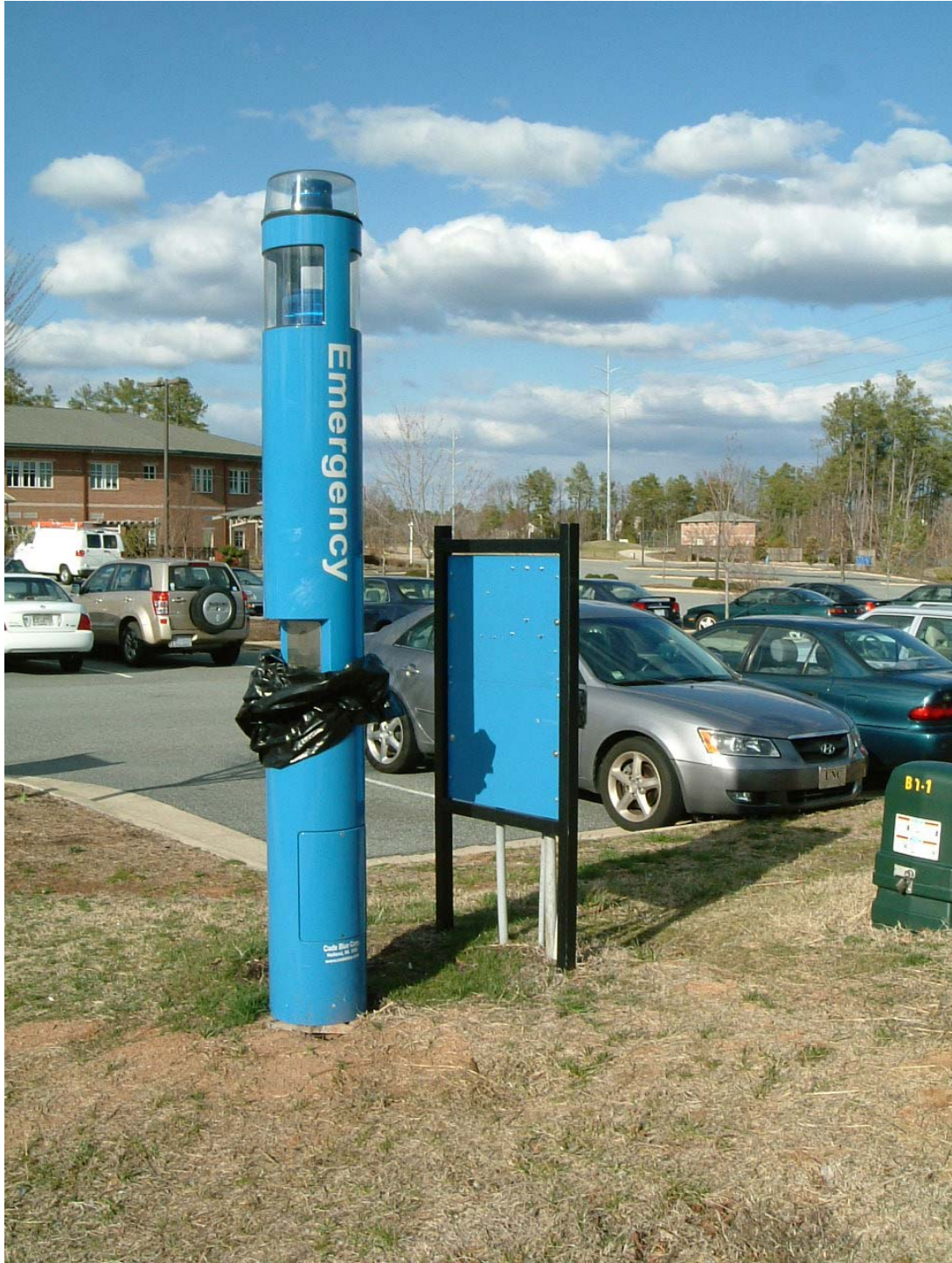
Photo 5: Emergency call station. It is not clear if it is operating.
