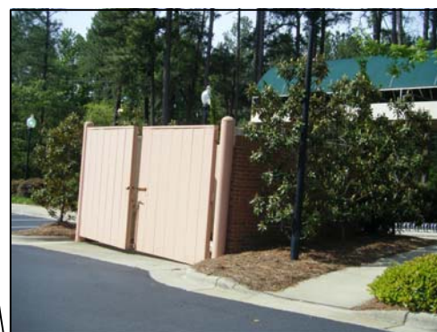
BOYD HALL DUMPSTER
