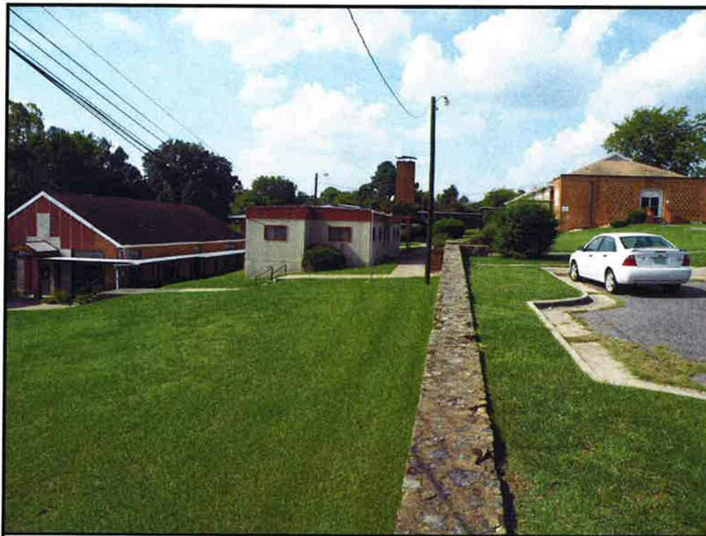
3 OF THE 4 TOTAL EXISTING BUILDINGS ON SITE AND STONE RETAINING WALL
