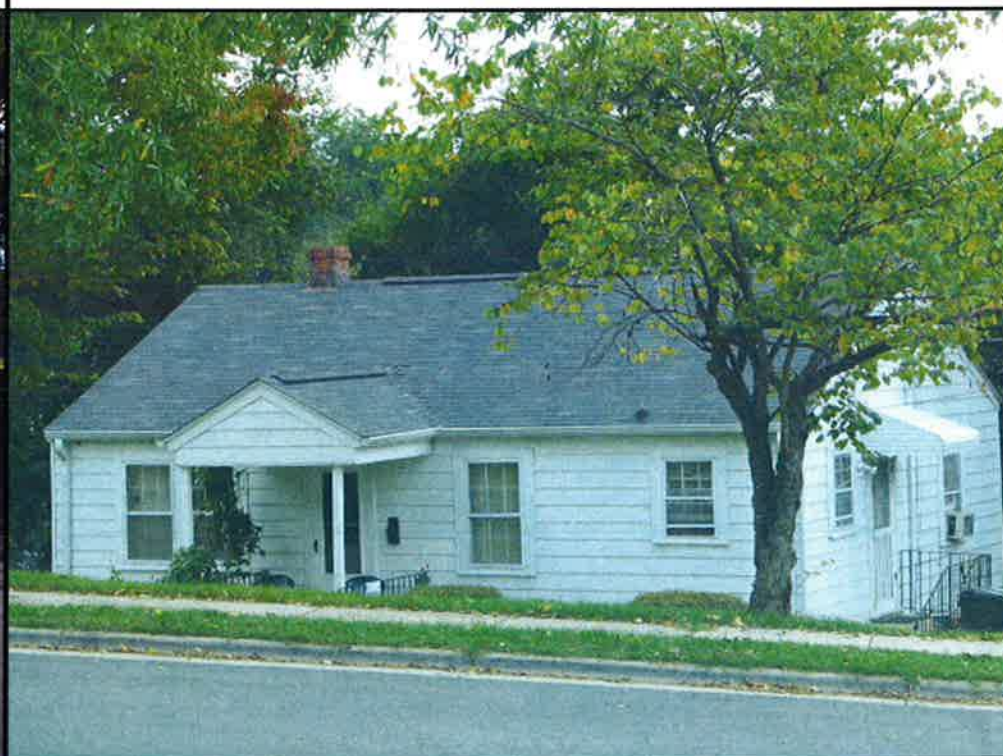
MANY ADJACENT HOUSES ARE ONE STORY RENTAL PROPERTIES
