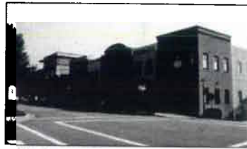
VIEW 11 400 BLOCK, NORTHEAST OF SITE
