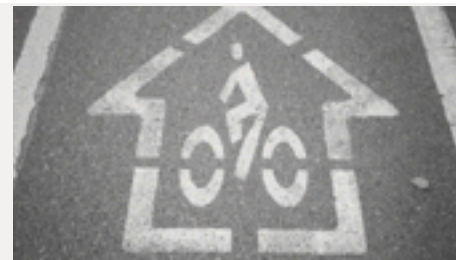
Denver’s innovative bike arrow is being used in many cities to help motorists and bicyclists share the road.
