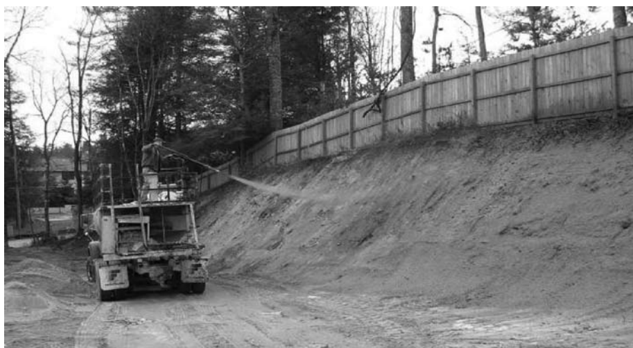
Figure 3. Seed, PAM, and a fiber mulch are applied to a steep slope with a hydroseeder.
