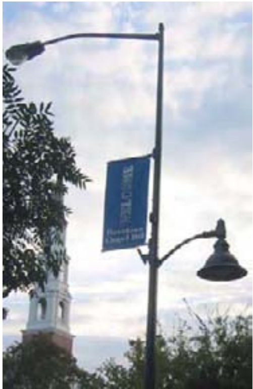
Chapel Hill’s standard Lumec Domus light fixture can be retrofitted with LED lights, a new and highly energy efficient option.
