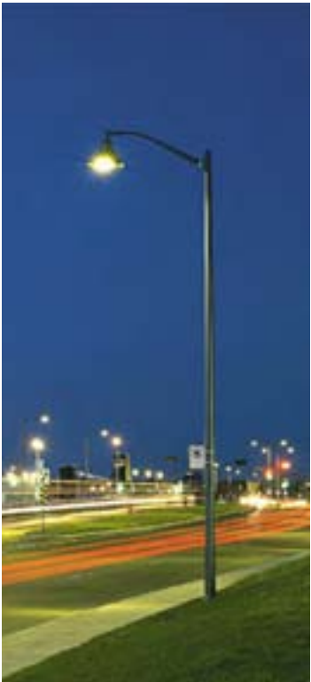
Chapel Hill’s standard Lumec Domus light fixture can be retrofitted with LED lights, a new and highly energy efficient option.
