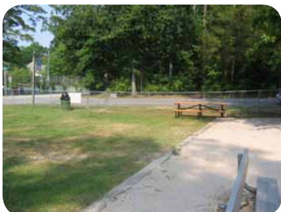
4 Older site furnishings should be replaced. New benches, waste receptacles and ADA accessible picnic tables need to be installed along an ADA accessible route.
