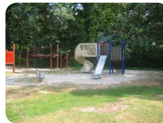
3 The safety surfacing needs to be removed and replaced with engineered wood fiber or poured-in-place rubber surfacing. Edging should be installed to ensure adequate safety surfacing remains within the fall zone.
