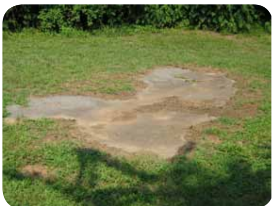
4 Areas such as this pavement should be removed from the greenway corridor, particularly since it is in the floodway of Bolin Creek. Pavement such as this is not usable, increases the impervious surface within the floodway, and is not aesthetically pleasing.
