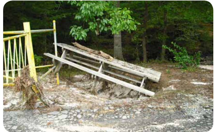
Image of flood damage after Hurricane Hannah during the summer of 2008. Photo courtesy of the Town of Chapel Hill.
