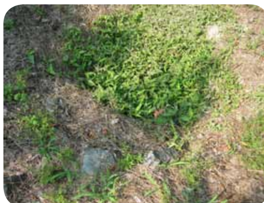
2 Clogged drainage pipes and culverts are increasing flood-related issues along this trail, including the deposits of sediment and leaf litter along the trail's surface.
