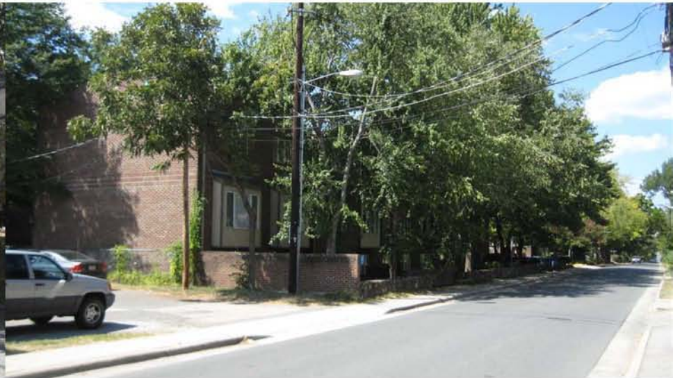
View of apartments on Church Street
