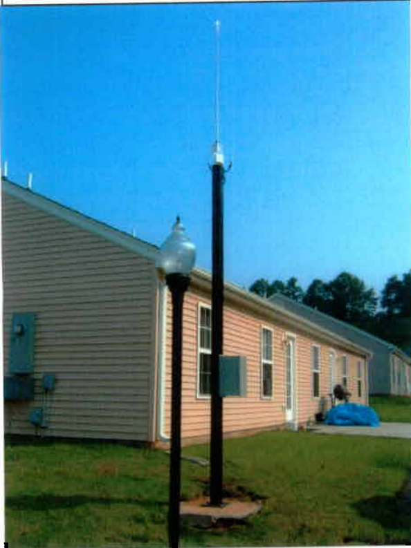
(A) Examples of ClearSKY radio enclosure and antennas on its own pole. (<18' total height)
