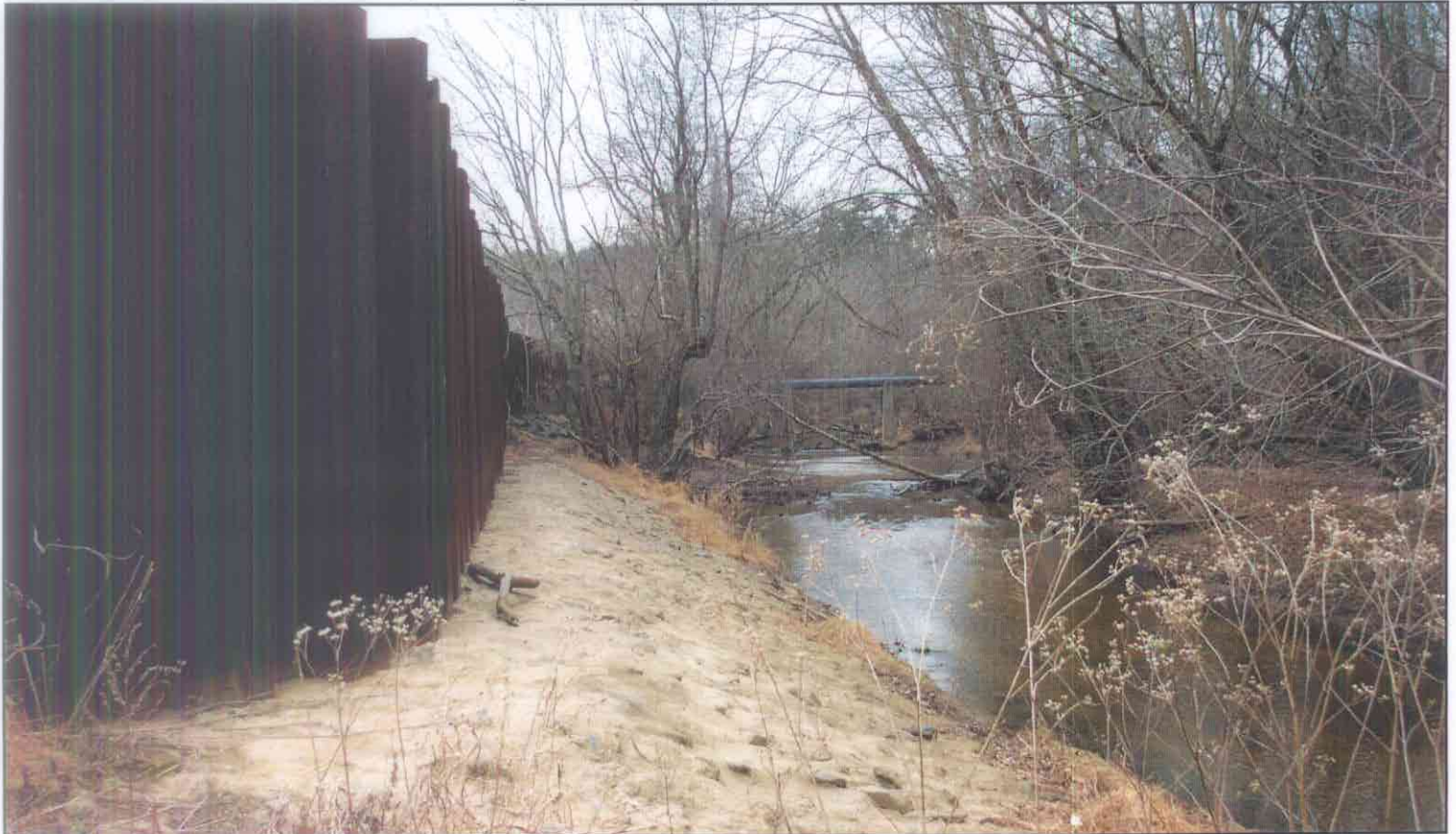
Hardened Steel Flood Protection, Looking North up Morgan Creek
