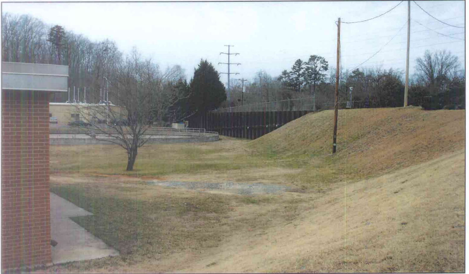
Earthen and Hardened Steel Flood Protection Berms Enclosing Mason Farm Treatment Plant, Looking Southeast
