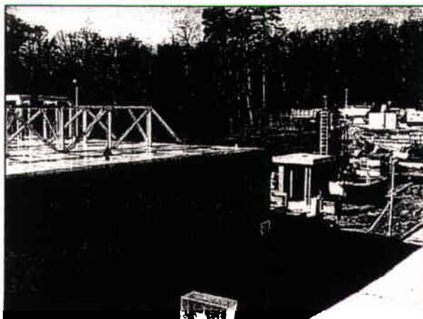
New covers installed in October, 2003 over the biosolids storage tanks.
