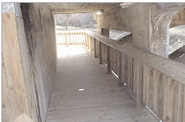
The extensive use of wood made the structure strong, practical, inexpensive, and aesthetically pleasing.
