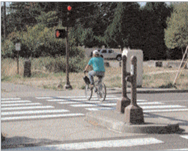
A pedestrian-activated signal button in a refuge island.
