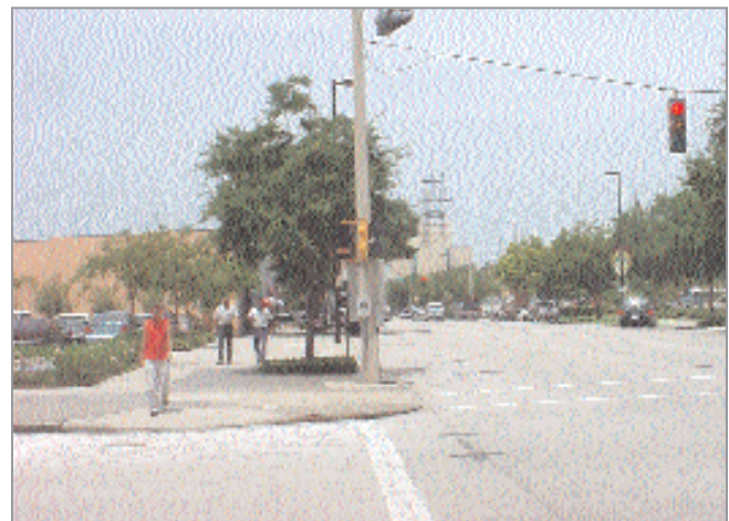
Pedestrians are given a WALK signal three seconds before parallel traffic is given a green light.
