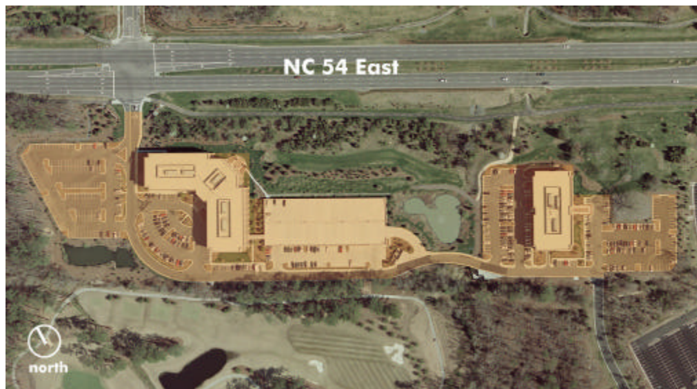
Figure 51 – Meadowmont Office Park
