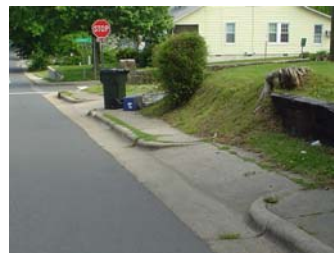
Church & Caldwell Street Trash and uneven sidewalk at driveway entrances.
